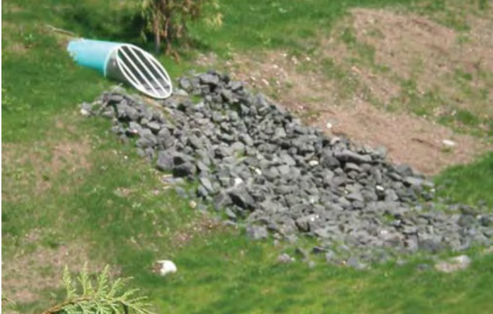
This energy dissipator is in good condition.
