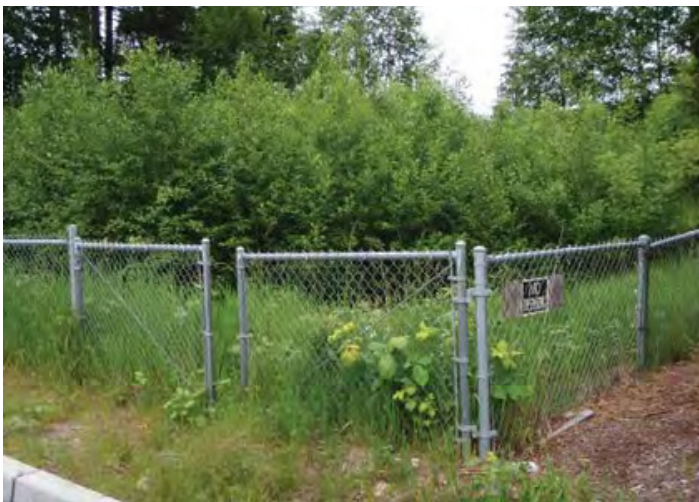
Alders and blackberry bushes have taken over this dry pond, hindering the infiltration of water.
